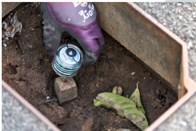
FIDO sensor installation.
