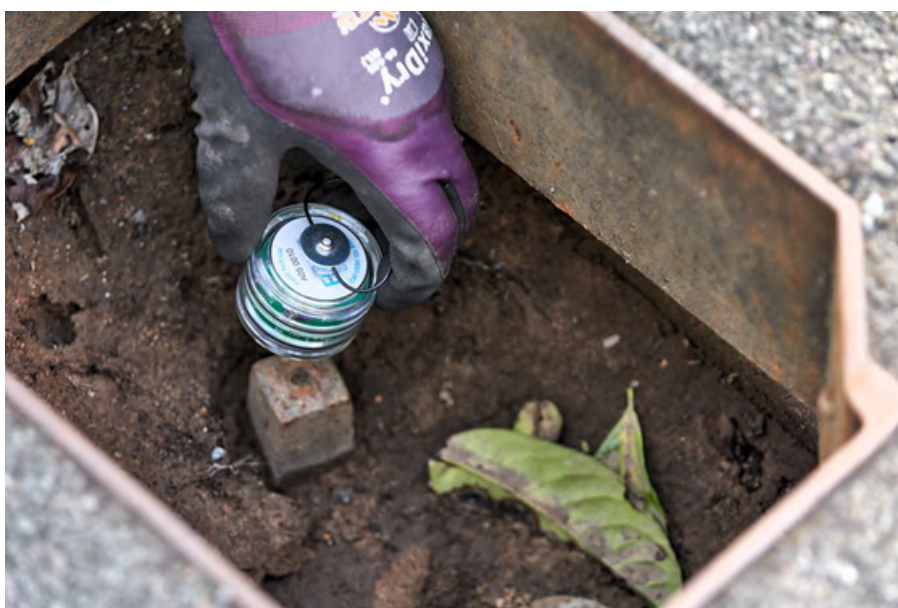
Installation of FIDO sensors.
